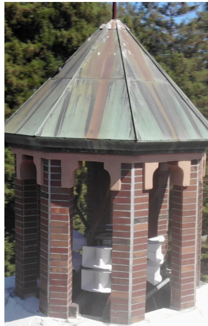
MILL VALLEY CITY HALL INSTALLATION
